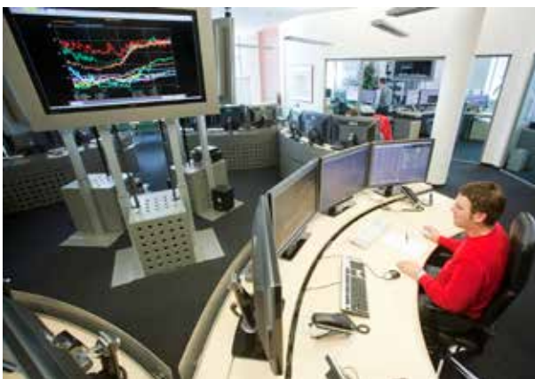
Network control centre of Avacon AG in Salzgitter.
